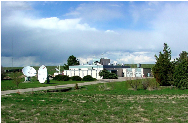
WWV transmitter building.
